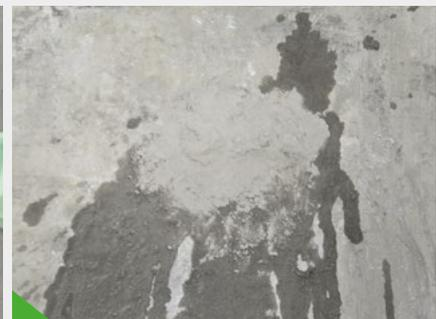
An active leakage is sealed instantly after applying KÖSTER KD 2 Blitz Powder.
