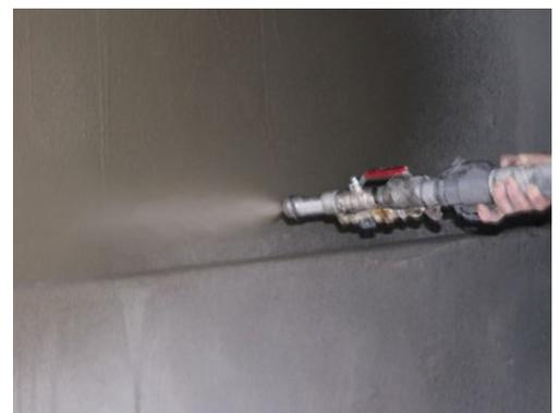
KÖSTER NB 1 Grey can either be applied with a brush or it can be sprayed onto the surface, e.g. with the KÖSTER Peristaltic Pump.
