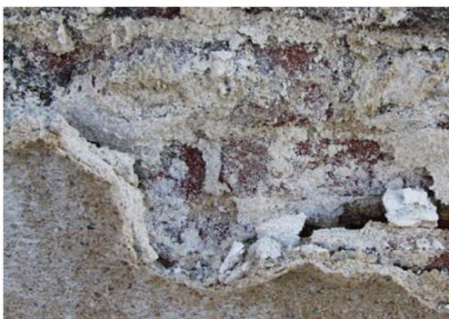
Typical damage through salt efflorescence.
