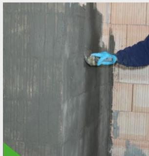
As negative side waterproofing, NB 1 Grey is generally applied in two layers.
