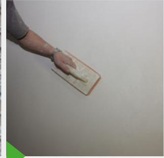
KÖSTER Restoration Plaster is applied to the fully cured key with a trowel or suitable spraying equipment. The surface is then floated smooth.
